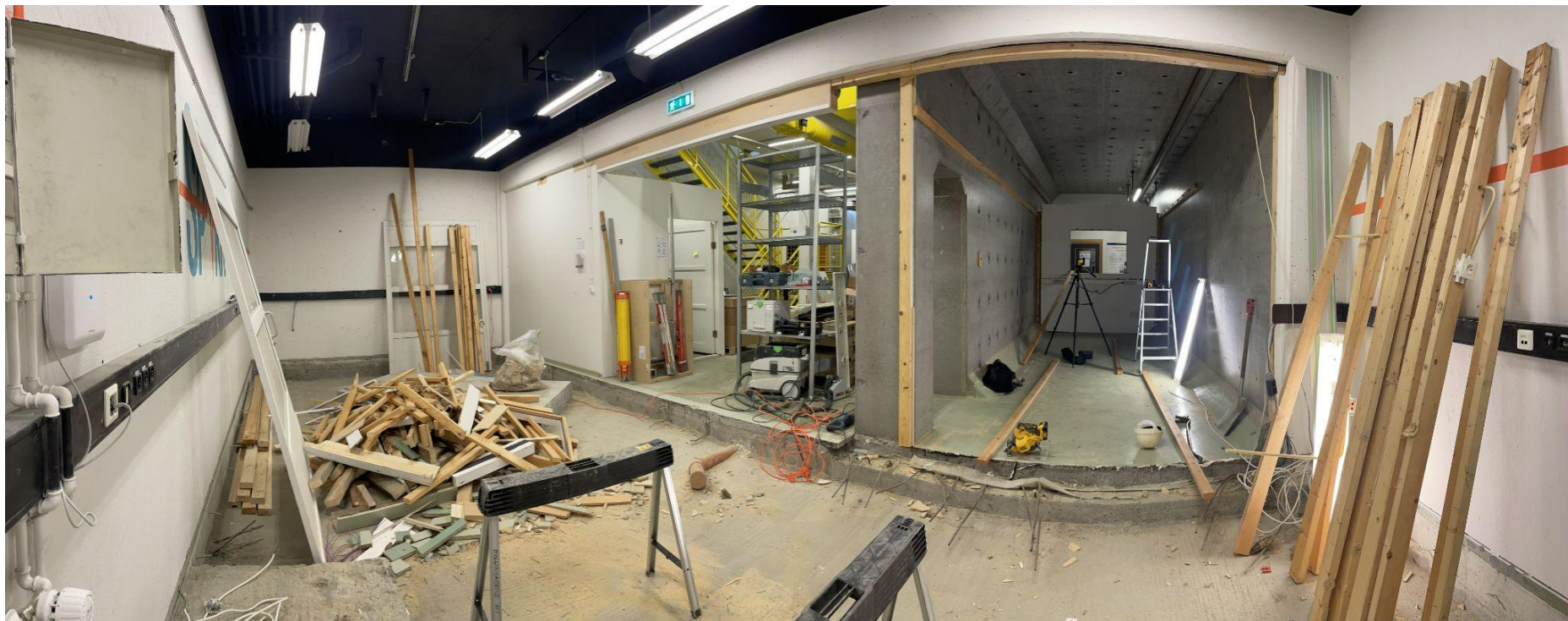
VR III lab space under construction
